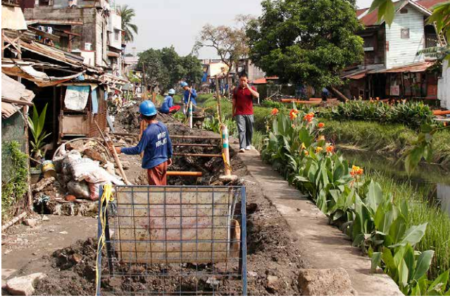
⌞ During construction of sewerage network
