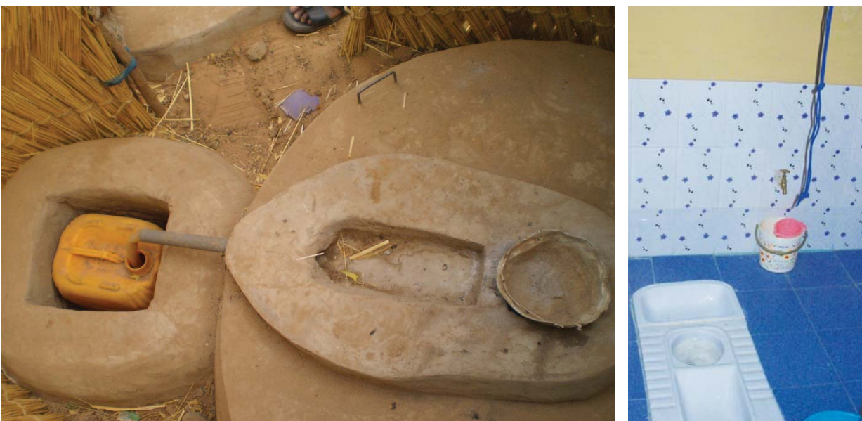
Urine-diverting composting toilet in Niger (left) and a demonstration urine-diverting toilet at the Tarumitra Bio-reserve and Ecology Centre, Bihar, India (right), with rope to facilitate use. Photos: Linus Dagerskog, Kim Andersson.
