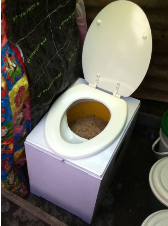
PHOTO 1 CBS toilet used in study
