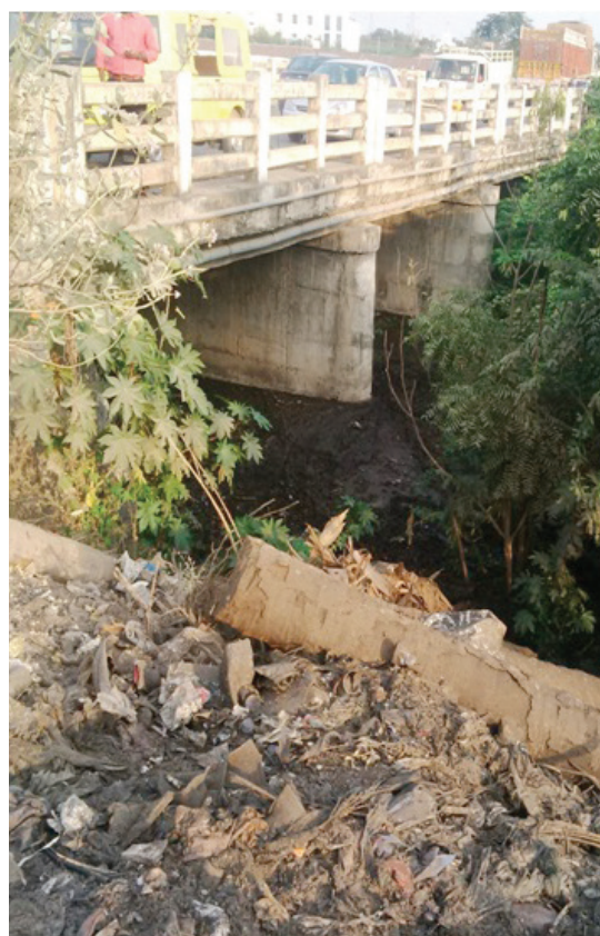
Septage disposal point at Alankar bridge
