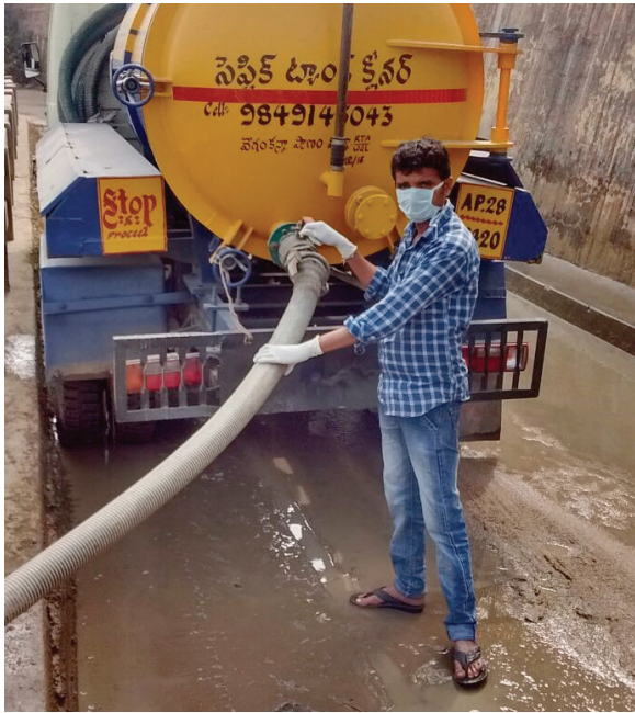
Figure 6: Licensed operator with an emptying vehicle truck
